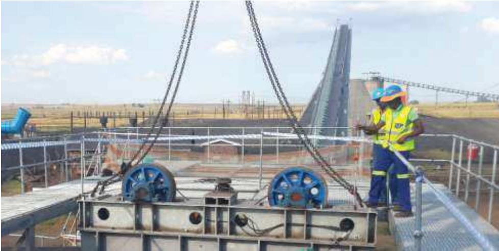
Civil works prepared up front
