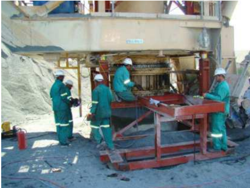
Lifting used to position the slew bearing in place
