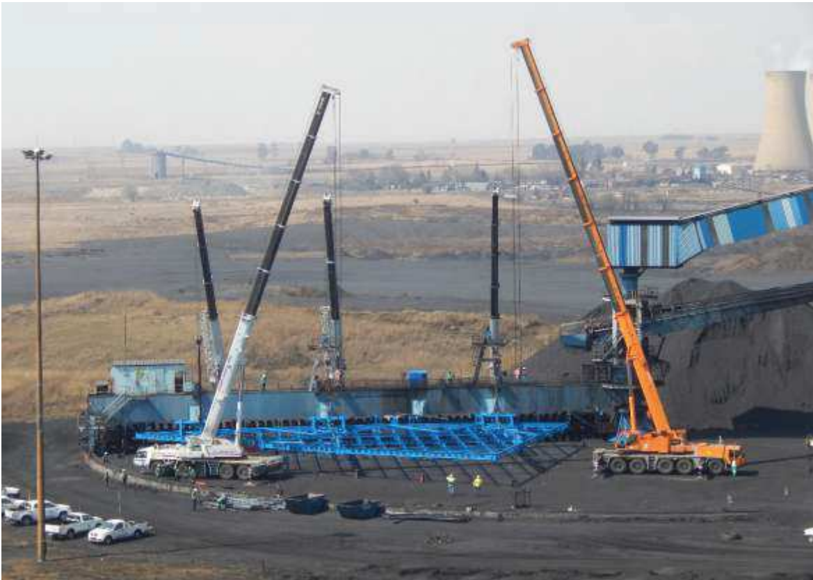
Tandem Lifting Used To Place Harrow
