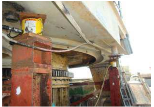
Slew Bearing replacement in Venetia diamond mine.
